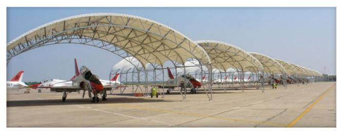
Shelter Structures is proud to announce that we have completed the design, manufacture and erection of 36 military hangars for the US Navy. The <u>aircraft hangars</u>, 50 feet long, 57 feet wide and 23 feet high, are protecting the Navy's T-45 Goshawk trainers. These aircraft are used in the final phase of training Navy pilots to land on aircraft carriers.
