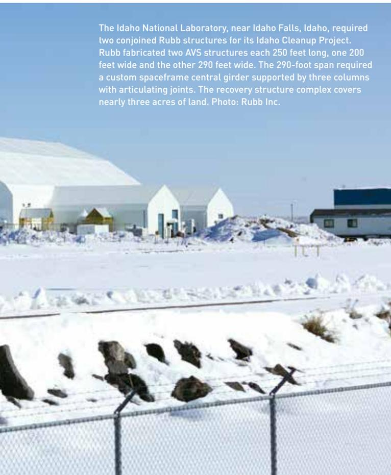
The Idaho National Laboratory, near Idaho Falls, Idaho, required two conjoined Rubb structures for its Idaho Cleanup Project. Rubb fabricated two AVS structures each 250 feet long, one 200 feet wide and the other 290 feet wide. The 290-foot span required a custom spaceframe central girder supported by three columns with articulating joints. The recovery structure complex covers nearly three acres of land. Photo: Rubb Inc.
