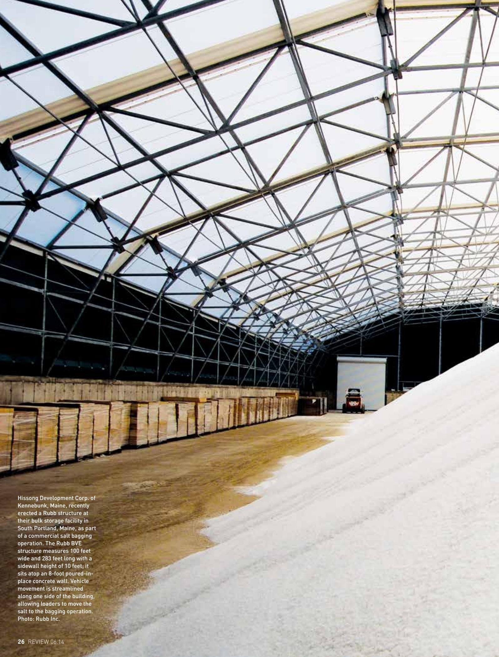
Hissong Development Corp. of Kennebunk, Maine, recently erected a Rubb structure at their bulk storage facility in South Portland, Maine, as part of a commercial salt bagging operation. The Rubb BVE structure measures 100 feet wide and 283 feet long with a sidewall height of 10 feet; it sits atop an 8-foot poured-in-place concrete wall. Vehicle movement is streamlined along one side of the building, allowing loaders to move the salt to the bagging operation. Photo: Rubb Inc.
