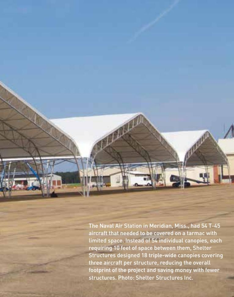
The Naval Air Station in Meridian, Miss., had 54 T-45 aircraft that needed to be covered on a tarmac with limited space. Instead of 54 individual canopies, each requiring 10 feet of space between them, Shelter Structures designed 18 triple-wide canopies covering three aircraft per structure, reducing the overall footprint of the project and saving money with fewer structures. Photo: Shelter Structures Inc.
