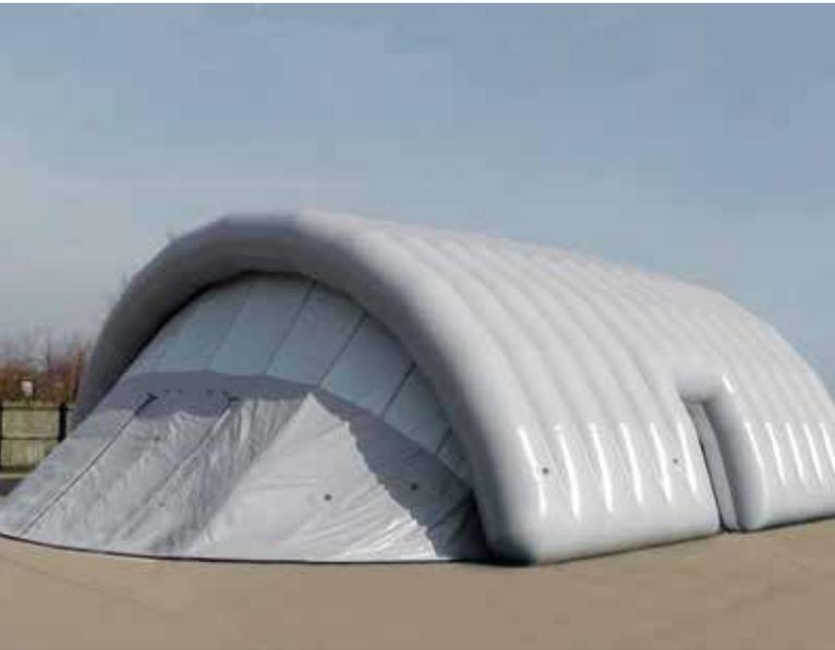
This portable hanger, designed and manufactured by Tectoniks Ltd., utilizes an air-inflated fabric structure technology of air tube beams, typically with spans up to 65 feet (20 meters); because it has a modular construction, it can be made any length. A variety of end terminations—fully inflated walls to membrane ends—can be used to create closure, as well as functioning door ends that can be opened for full-width access. Photo: Tectoniks Ltd.
