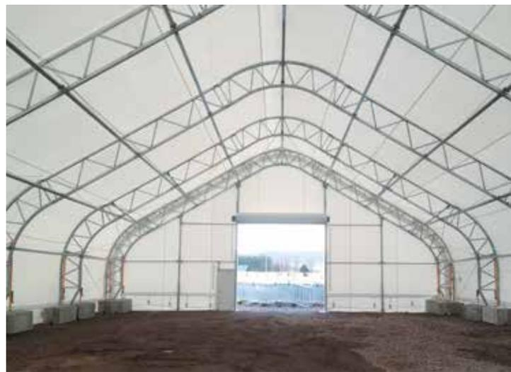
When challenged with locating structures on unpredictable surfaces, Shelter Structures uses its ballast system that enables a shelter to be securely anchored without the use of foundations or earth anchors. The heavy-weight system shortens the time needed to install and allows rapid redeployment when moved. Photo: Shelter Structures Inc.
