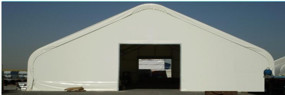
This steel framed fabric covered structure is 60 feet wide and 100 feet long with overhead metal doors as access for temporary warehouse storage.
